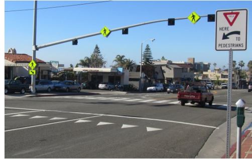
Pedestrian signage and flashing beacons along Coast Highway
