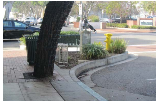
Curb extension in Laguna Beach
