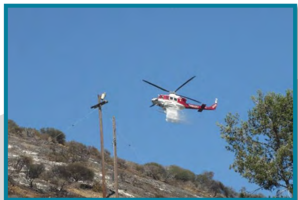
2012 Transformer/Pole Fire between Coast Hwy. and Nyes Place
