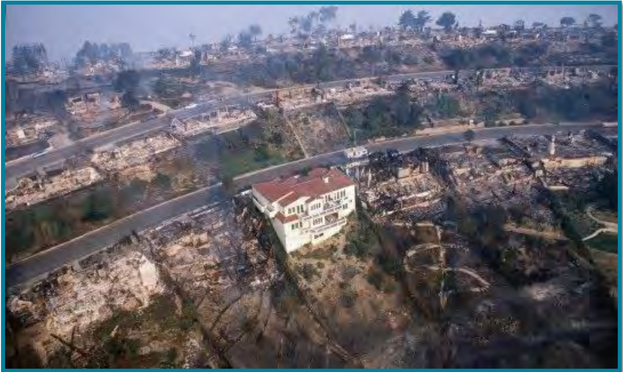
Fire resistant home survived 1993 Laguna Fire, Skyline-Tahiti neighborhoods
