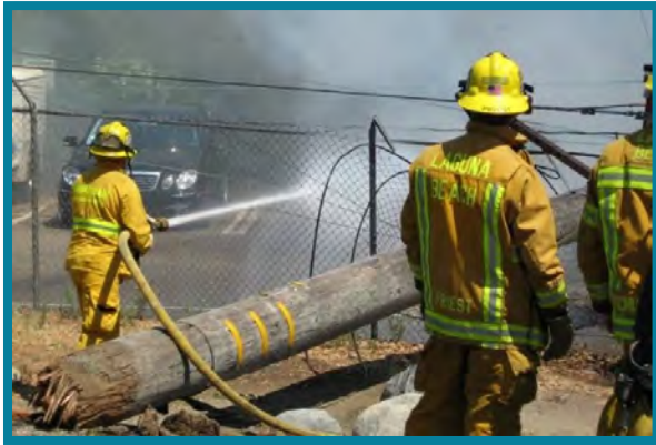
2007 Laguna Canyon Road Transmission Pole / Fire
