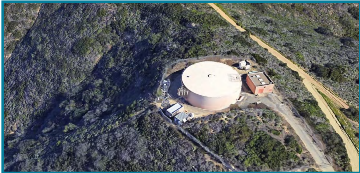
Antennas on Ridge Reservoir
