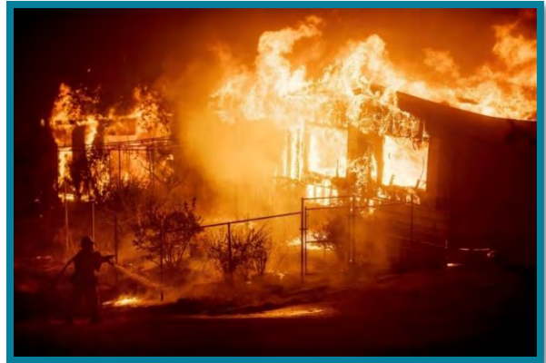
Structural loss to the Camp Fire City of Paradise, 2018
