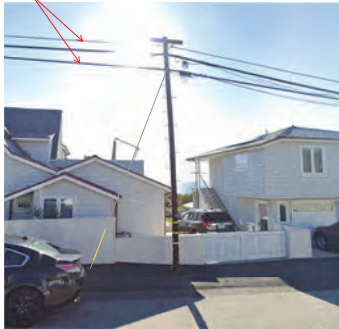
Ex. Wires to be Removed
