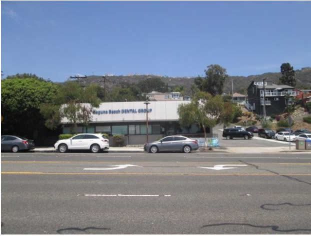
1. View of the Site from the west.
