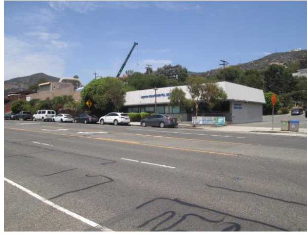
2. View of the Site from the southwest.
