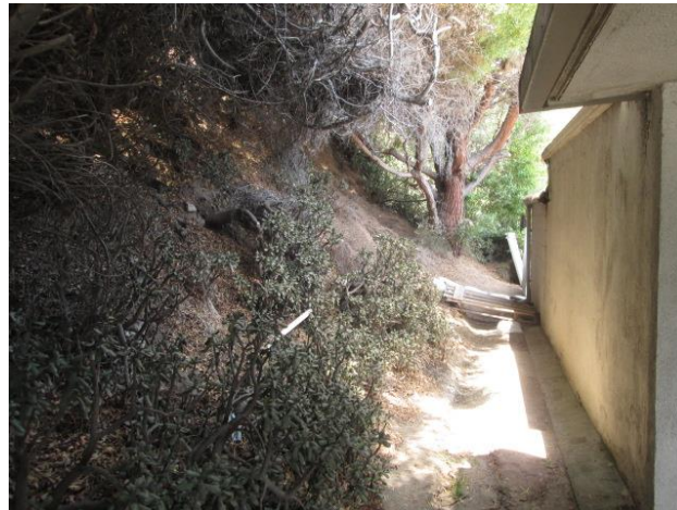
5. Northern side of building.
