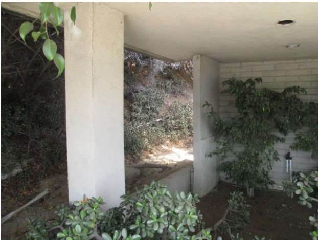
4. Northwest corner of building.
