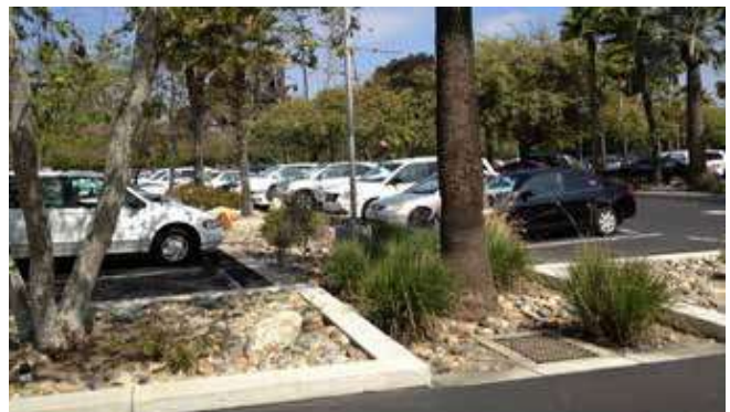
Parking lot with stormwater planters.
