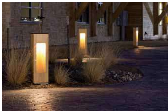
Lighting in parking lots should be pedestrian oriented along walkways
