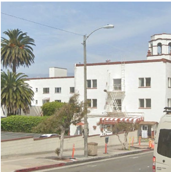
Coast Highway near Hotel Laguna (overhead wiring)
