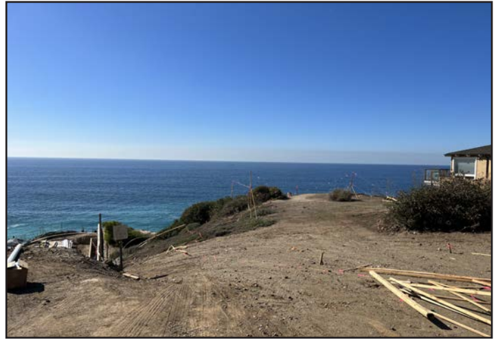
View 2: View looking southwest from Coast Highway across the Project Site.
