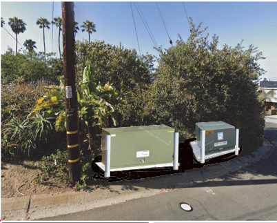
SDGE TERMINATOR CABINET 66" x 22" x 33" (DARK GREEN FINISH) W/ TWO BOLLARDS SDGE PAD-MOUNTED TRANSFORMER 36" x 33" x 26" (DARK GREEN FINISH) W/ TWO BOLLARDS
