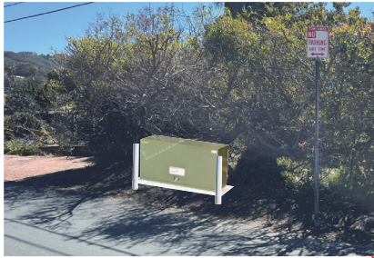
SDGE TERMINATOR CABINET 68" x 22" x 33" (DARK GREEN FINISH) W/ TWO BOLLARDS
