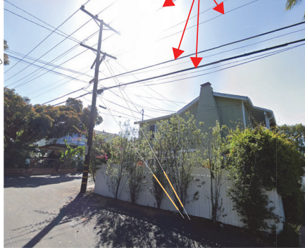
GUY ANCHORS AT RISER UTILITY POLE
