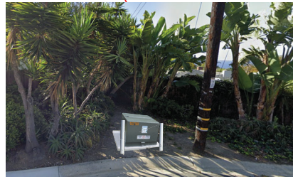
SDGE PAD-MOUNTED TRANSFORMER 36" x 33" X 26" (DARK GREEN FINISH) W/ TWO BOLLARDS
