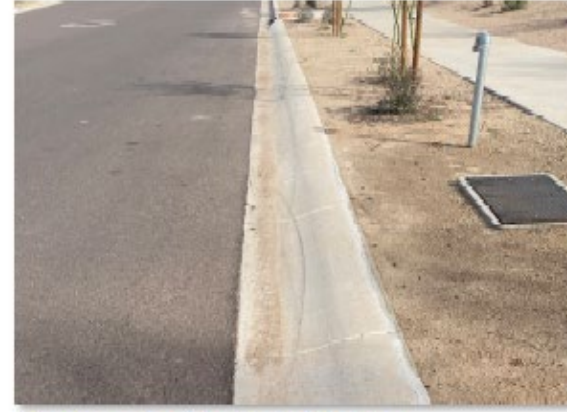
Concrete Rolled Curbs
