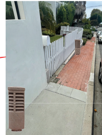
SCE VENT STANDPIPES 10" DIAMETER, 34" HEIGHT SANDSTONE (BROWN) FINISH
