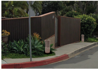
SCE VENT STANDPIPES 10" DIAMETER, 34" HEIGHT SANDSTONE (BROWN) FINISH
