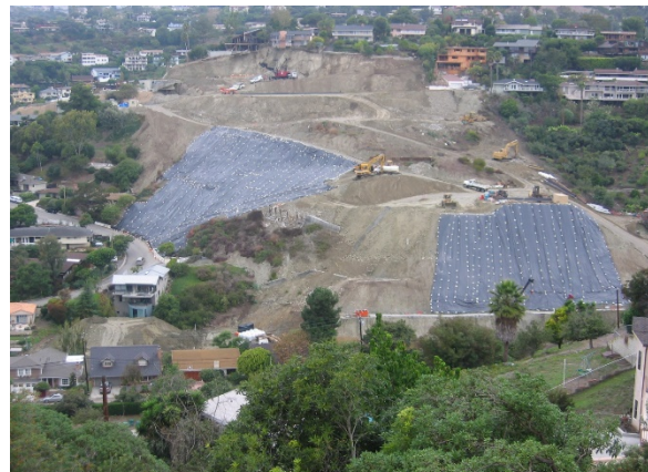
Remediation work from the 2005 Bluebird Canyon Landslide.
