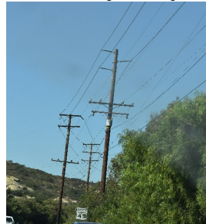
Example of overhead powerlines
