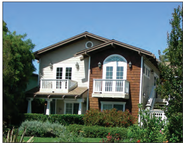
The combination of materials on this façade provides architectural detail that reduces the perceived mass.
