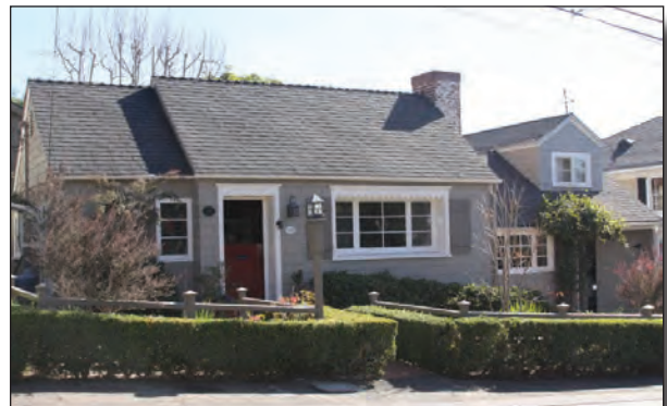
The additions and modifications to this 1935 historic residence were designed to preserve its historically significant features, including windows, doors, chimney and materials.
