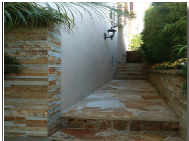
The stonework matches the hardscape and terminates at a logical point (away from the immediate public view).
