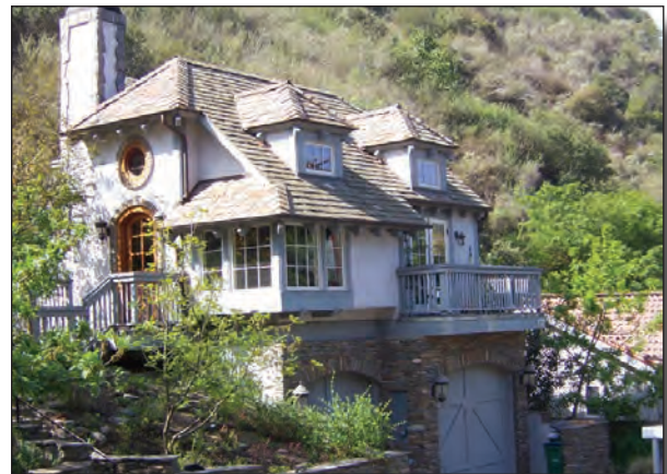
This home is built in a fuel-modification zone with fire-resistant materials like stone, stucco and tile.
