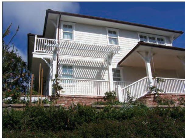
The simple building form of this residence is enhanced with the trellis, covered porch, variation in building materials, balcony, extended eaves and window trim.
