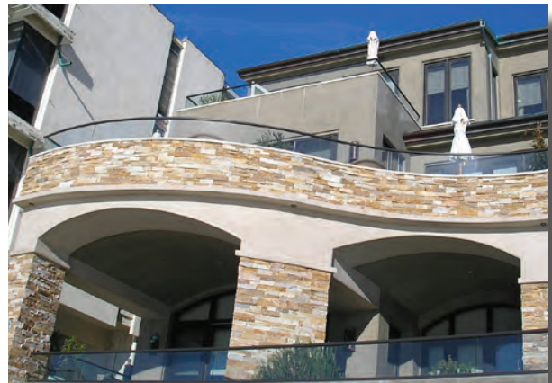
Natural stone, stucco and metal capped glass railings were selected on this oceanfront home to withstand the harsh coastal environment.
