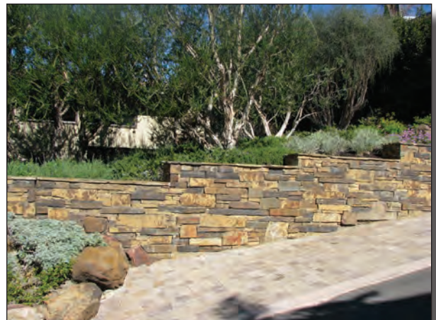
These retaining walls were designed to follow the site topography in effort to minimize their visual impact.
