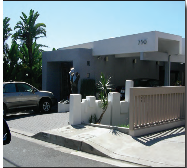
Single-car garage with adjacent carport. The enclosed garage could be designed as a tandem configuration to allow parking for two cars.
